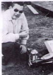
Still another MPC product: this MK pump powers the go-jack into task as author watches.
